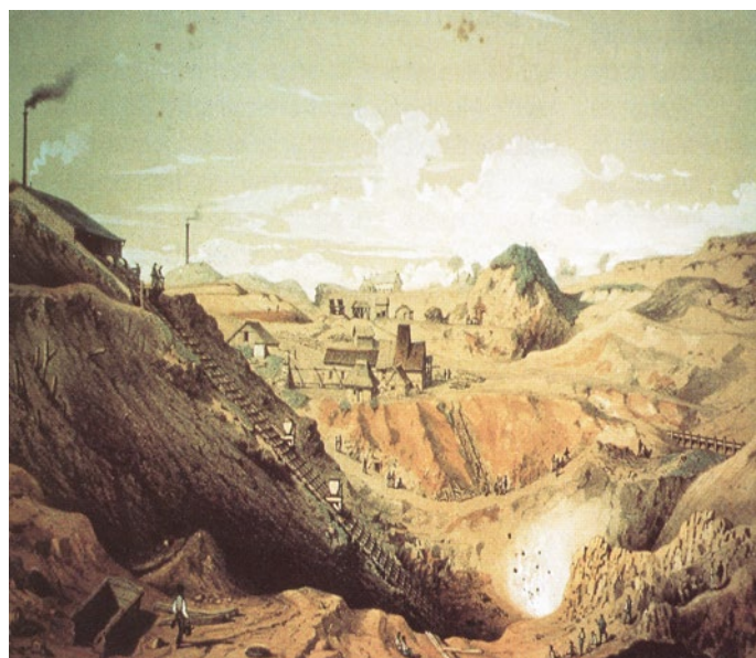
Fig. 2. — Engravings from Adolphe Maugendre, around 1850. La Calamine (Moresnet) deposit. General view of the processing plant (above) and of the north side of the open-pit exploitation (below). Source : Museum Vieille-Montagne (formerly Göhlthal Museum), La Calamine, photo Léon Dejonghe. Reproduced from Ladeuze et al. (1991).
